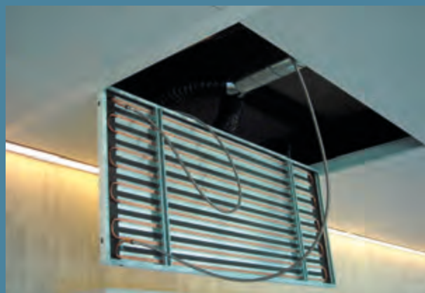
pannello metallico radiante chilled metal panel
