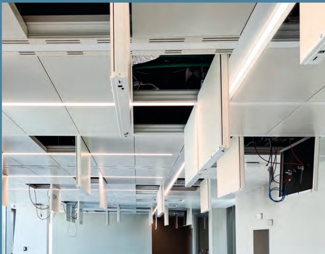
pannello metallico radiante chilled metal panel
